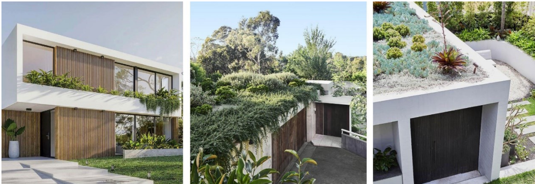
Example of planted roofs
