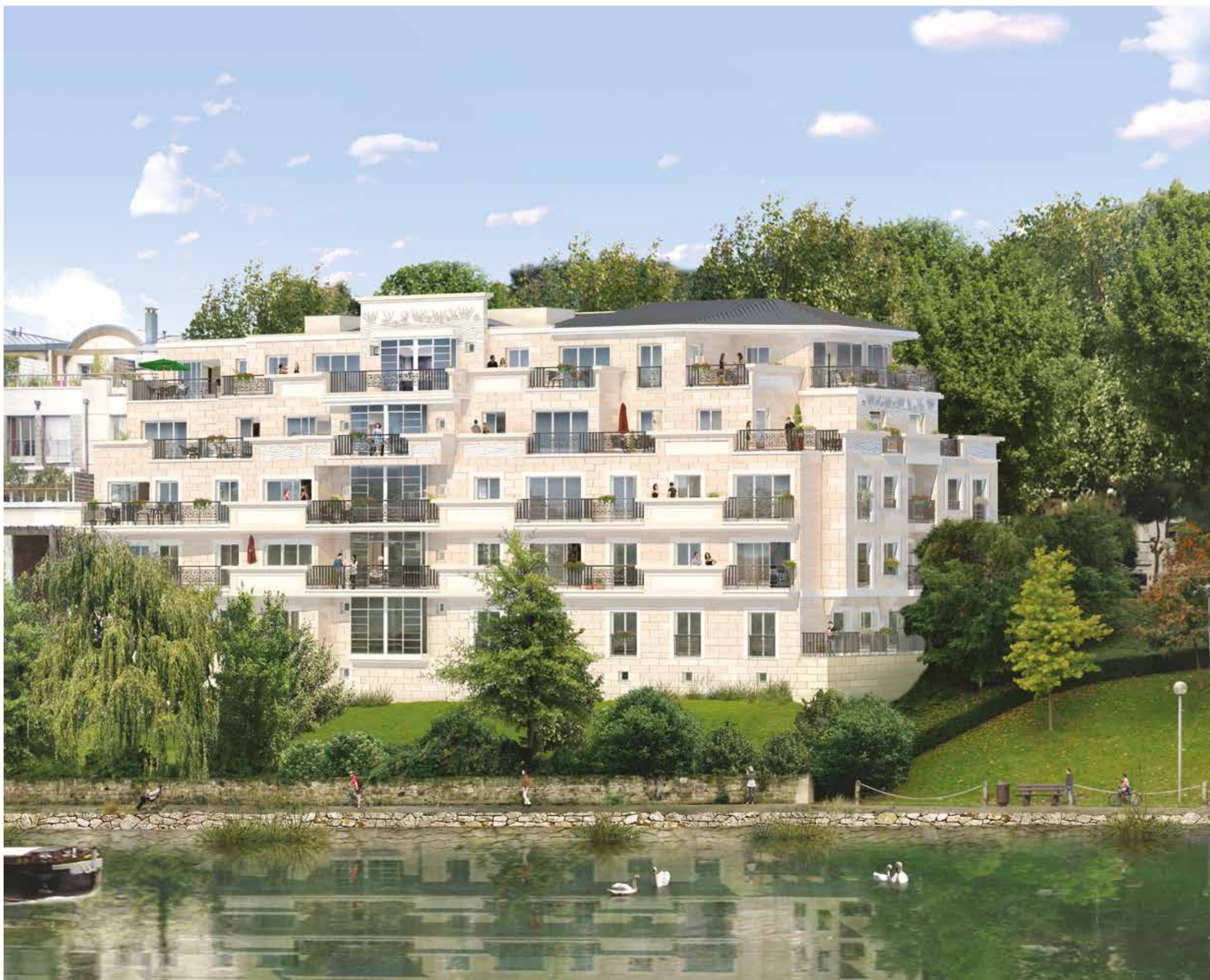
The Neuilly La Grande Jatte Residence viewed from the Seine.
